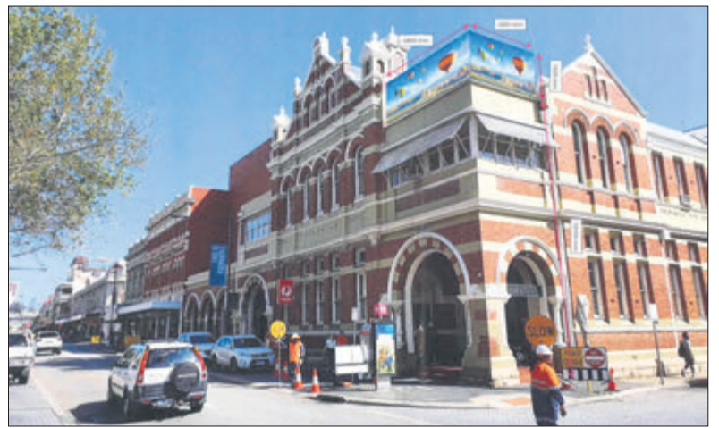
• Freo council has knocked back this proposed electronic billboard on the old Post Office.
