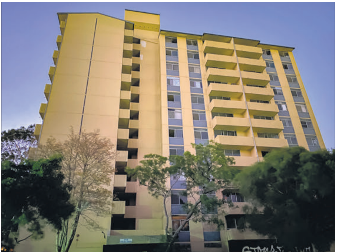
Stirling Towers have been empty near 10 years, and are a popular spot for urban explorers despite the security measures. Photo by www.streetkidindustries.com
