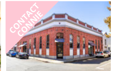
38/4/56 Pakenham Street, Fremantle
