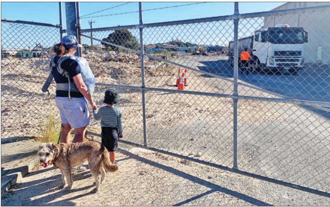
• Beaconsfield resident Lauren watches heavy machinery prepare the site for development, which she fears will lead to traffic problems. Photo by Steve Grant
