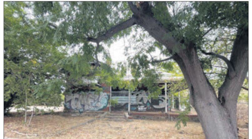
• The Guildford Road cottage is boarded up and in poor condition.
