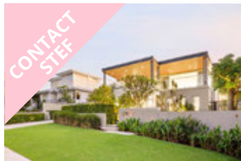
3 Chauncy Street, East Fremantle
